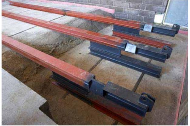
Check the level and position of the beams in relation to each other and to the boiler.
