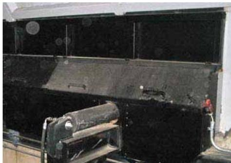
Install the stoker auger covers (6) and weld them to the hinges on the horizontal beams of the stoker partition.
