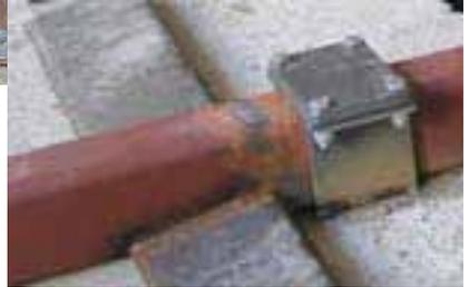
The bolts of the control tunnel cover should be pretightened before installation. Weld the control tunnels to the bottom beams in the concrete casting by the outer edges only, as shown in picture TPYM1003e.
