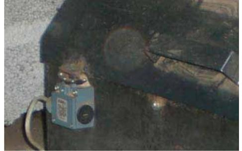
Fit the hopper cover and its frame hinge-side in the direction of the stoker. On the intermediate tank service hatch cover, install the limit switch that acts as a blockage monitor and the optical sensor that checks the fuel level (see picture). Connect these to the plant's automation system.
