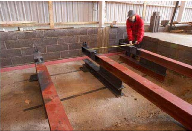
Place the edge beam in position. Weld it tight.
